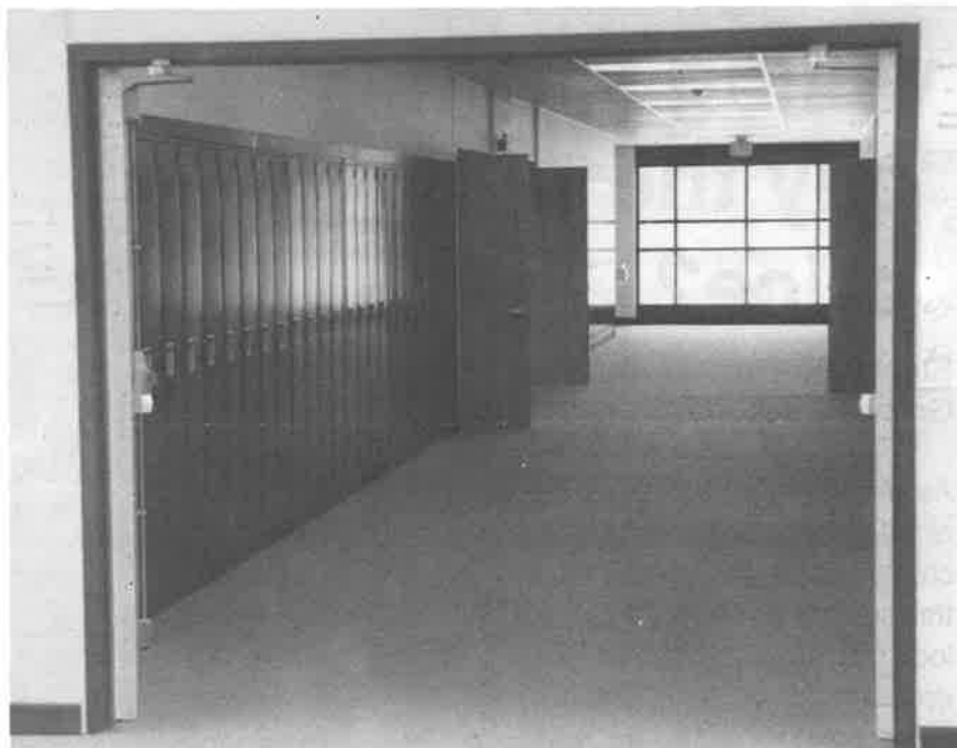
Here is the second floor finished product.
